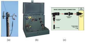
Figure 2. (a) Typical riser pole with overhead fuse cutout (3) Eaton single-phase pad-mounted transformer (c) Diagram of typical UG cable connection to transformer
